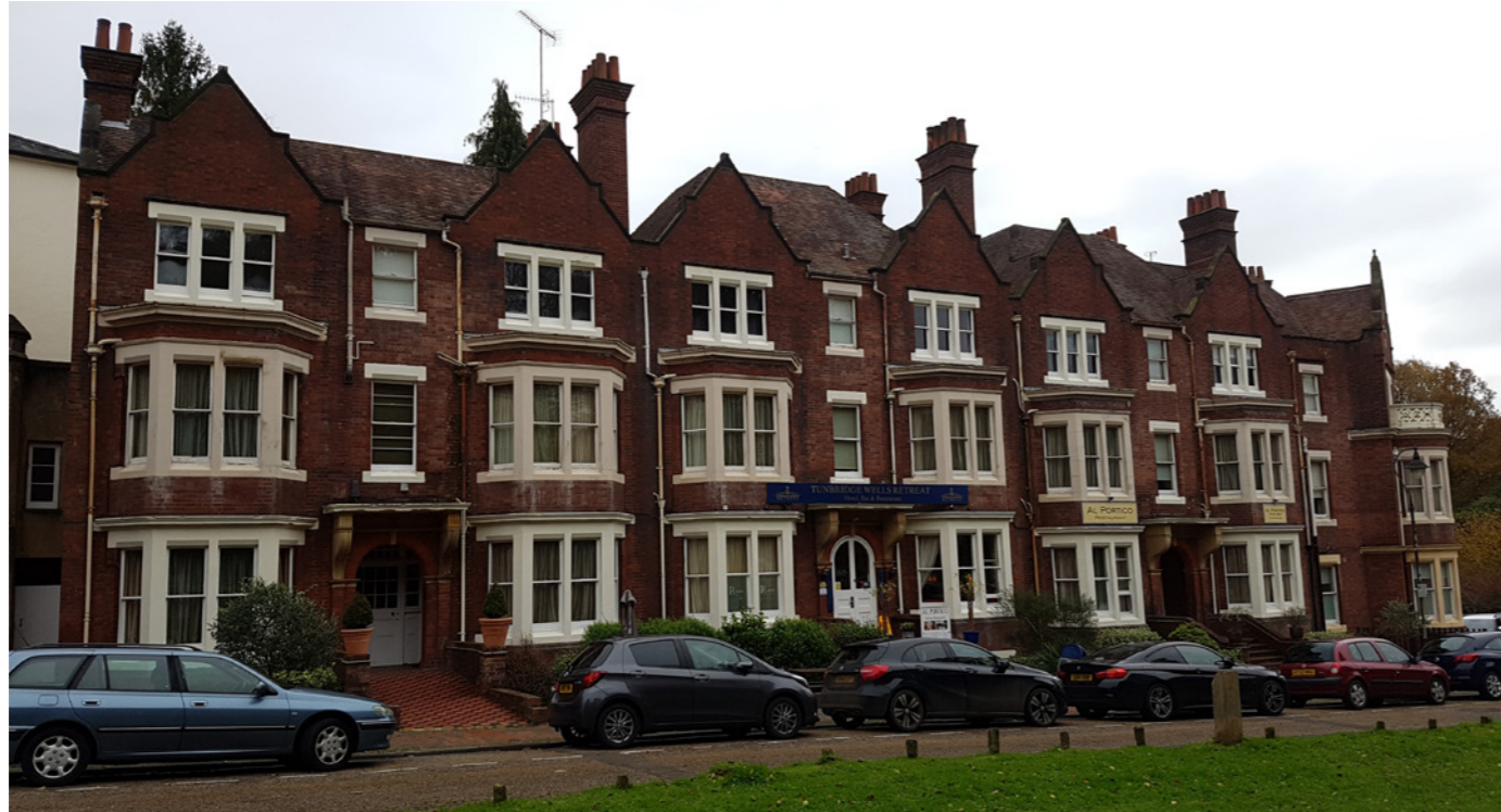
Photograph of West Elevation
