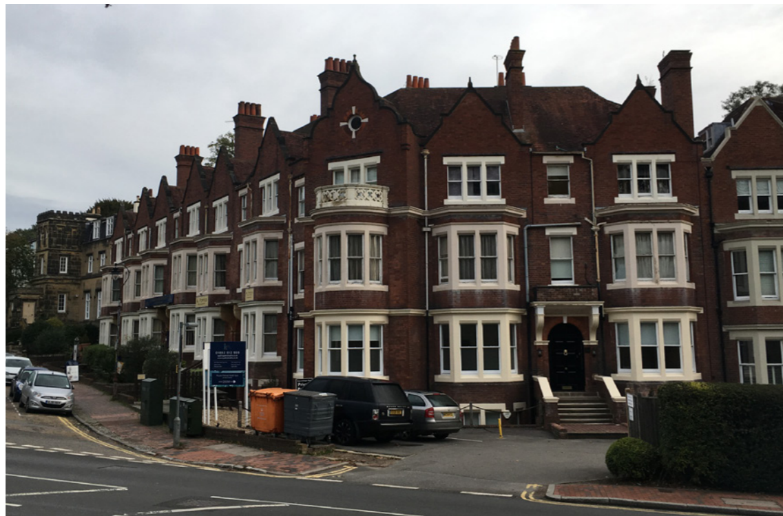
Photograph of South West Elevation (first floor and above)
