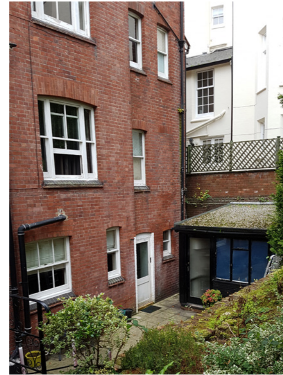
Photograph of Existing East/Rear Elevation
