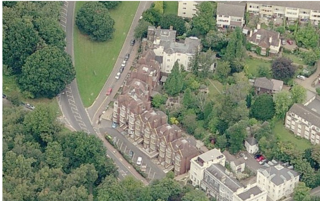
Aerial View of Site Looking North
